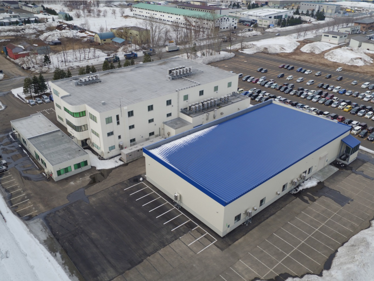
Blue roof of the new factory building (2nd factory). Seen behind is the existing 3-storied building.
