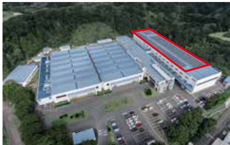
Solar power facility of Kikugawa Factory (Red flame)
