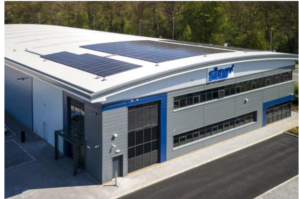
▲ Exterior of the building (aerial view)
